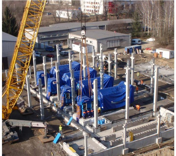
In early 2014 the four gensets were installed at the construction site in Tabor/Sezimovo Ústí
